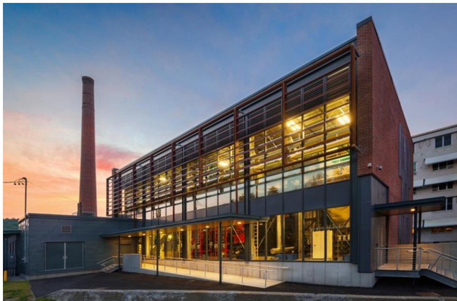
Capitol District Energy Plant - © Gary Hall Photography, courtesy GB Architects (GBA)
